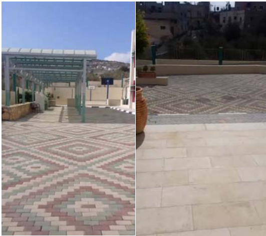
Fig.7. Paving the exterior fields using white stones and light blocks
