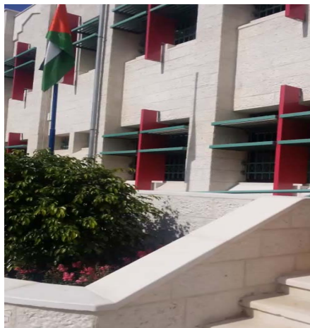
Fig. 3. Shading system on windows
